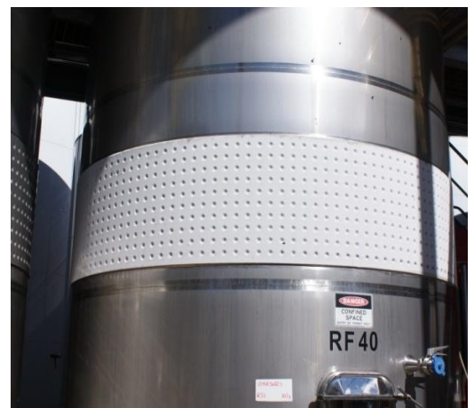
Figure 5: Iced up cooling jacket: No shade or insulation
