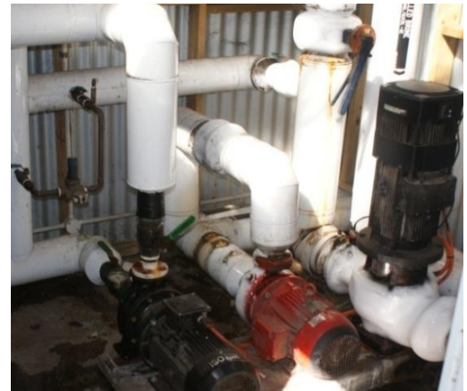
Figure 5: Iced up cooling jacket: No shade or insulation
