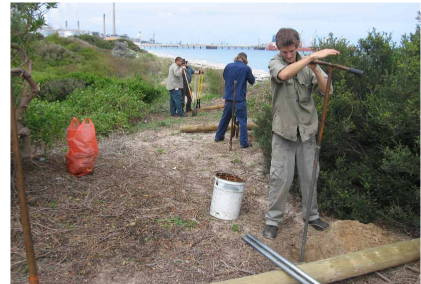
Green Jobs Corps trainees installing the access path fence.
